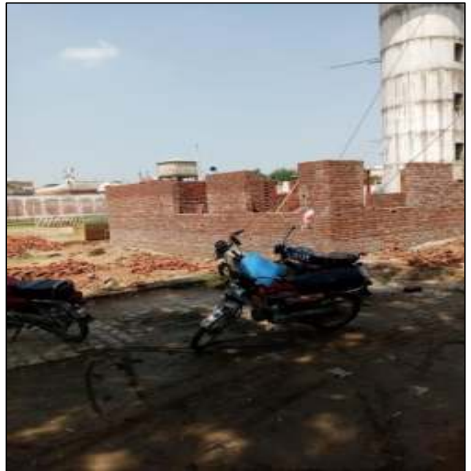
Picture 22: Construction of Servant Room
