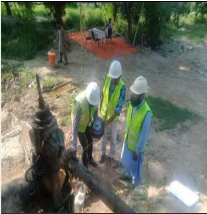
Picture 17: Pump out Test
