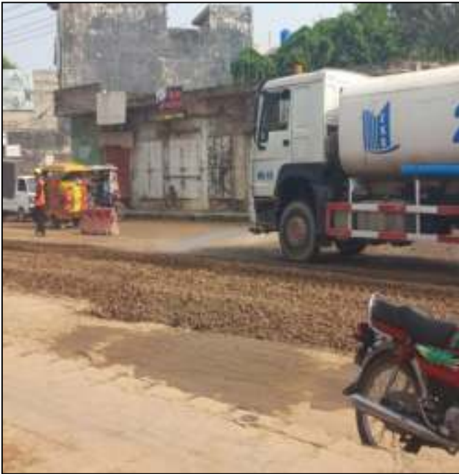
Picture 41: Spreading and Grading of Aggregate Base Course @ Defence Road
