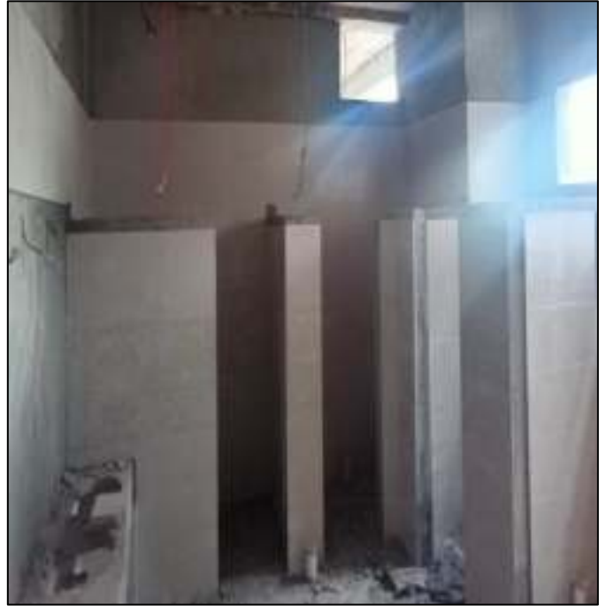
Picture 59: Porcelain Tile work in washroom
