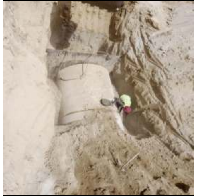
Picture 36: Jointing of 72" Dia Pipe
