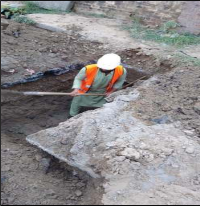
Picture 53: Excavation for laying HDPE pipe
