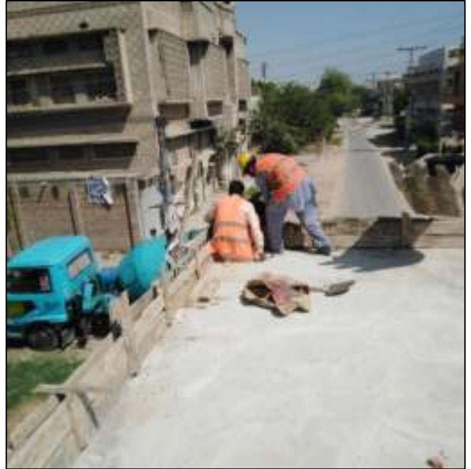
Picture 20: Shuttering of Parapet wall
