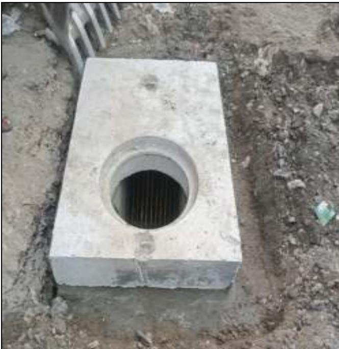
Picture 43: Grating Chambers Constructed @ Defence Road
