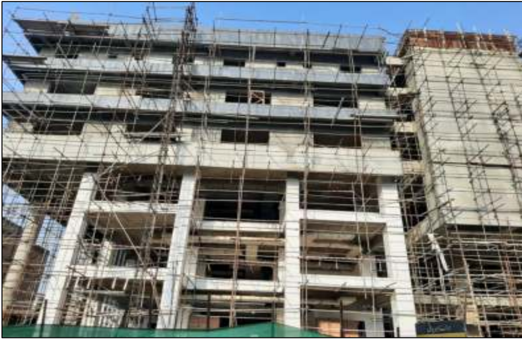
Picture 57: Cladding work on outer walls
