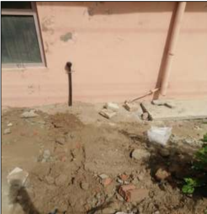
Picture 21: House connection for water supply pipe line
