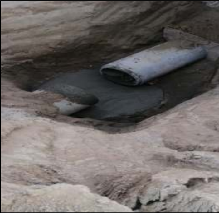
Picture 27: Laying of 42" dia pipe 1.9.5
