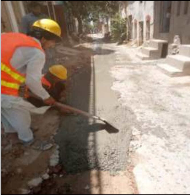
Picture 15: Restoration of PCC
