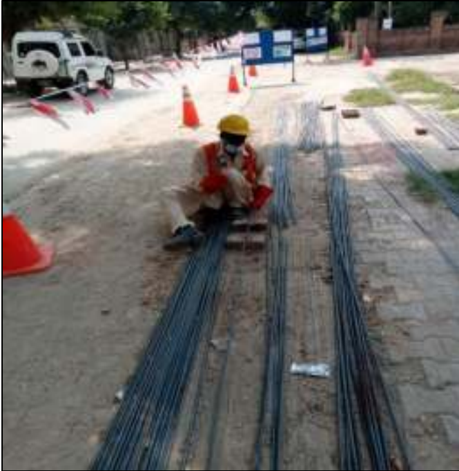
Picture 19: Steel Cutting of staff quarter for Roof
