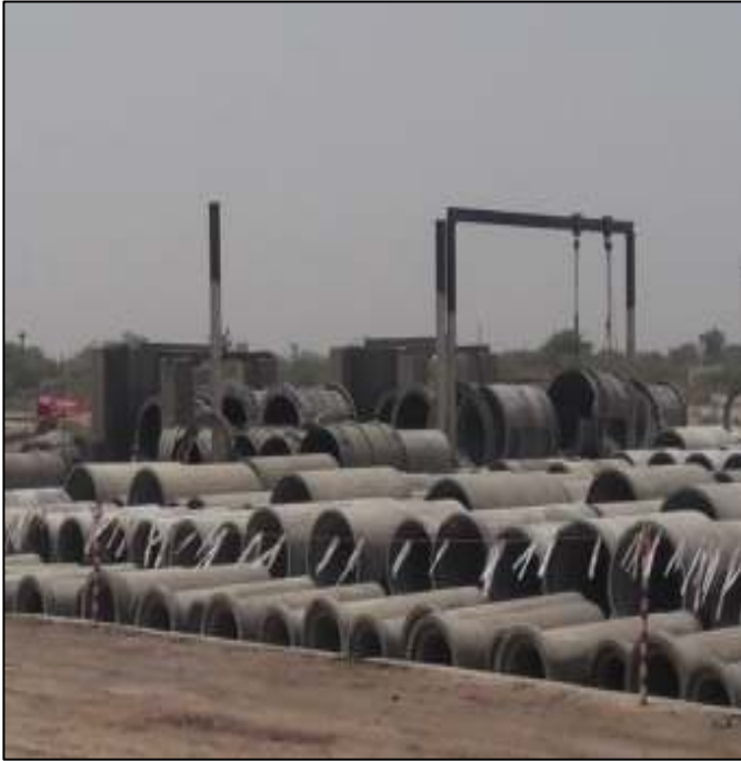
Picture 35: Curing of RCC Pipe at RCC Pipe Factory
