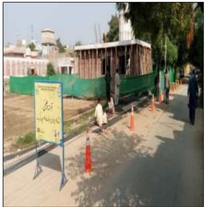
Picture 18: Steel Cutting of staff quarter for Roof Slab
