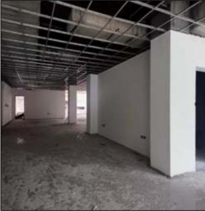
Picture 60: Paint work on walls of Ground floor
