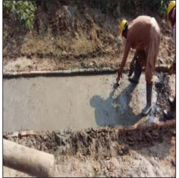
Picture 50: PCC in Foundation of Boundary Wall
