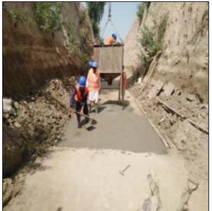
Picture 30: Concrete of Roof slab for Conduit
