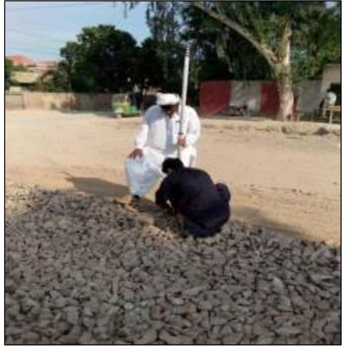
Picture 40: Survey Work is in Progress
