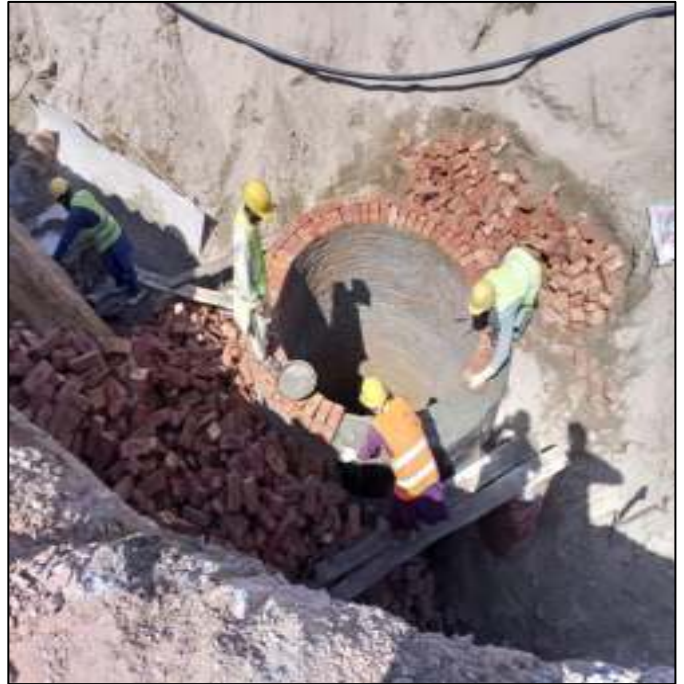
Picture 34: Construction of Manhole at 72' dia pipe line
