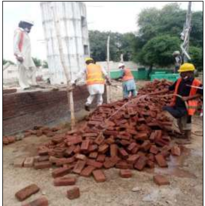
Picture 16: Brick work of Staff Quarter at T-05
