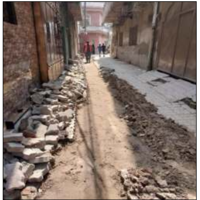
Picture 56: Restoration of Trenches in Progress in UC Muhammad Pura
