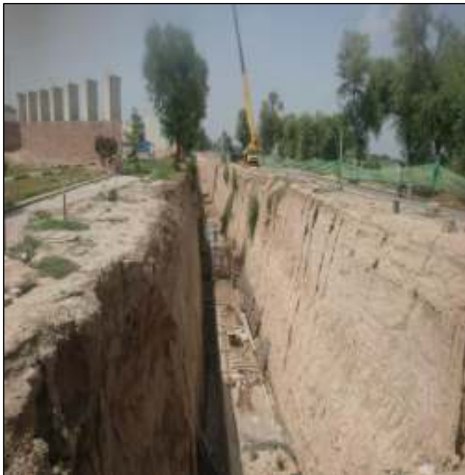
Picture 29: Excavation for conduit
