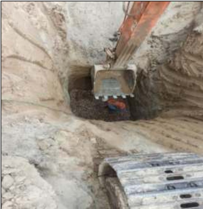
Picture 25: Laying of 48" dia L.2 Kacha Paka Noor Shah Road
