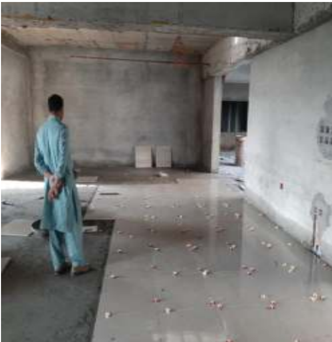
Picture 58: Tile work on 4th floor
