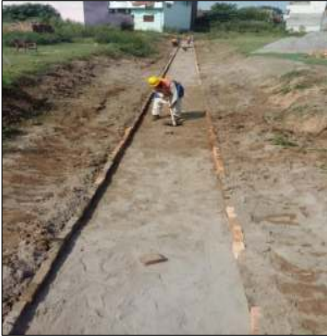
Picture 49: Bed Preparation for Laying PCC of Boundary Wall
