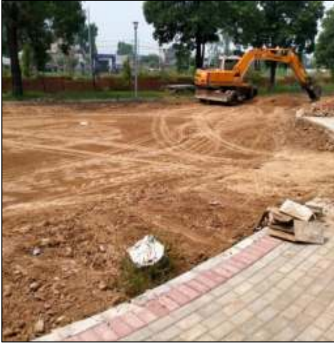
Picture 11: Clearing & Grubbing work in Progress
