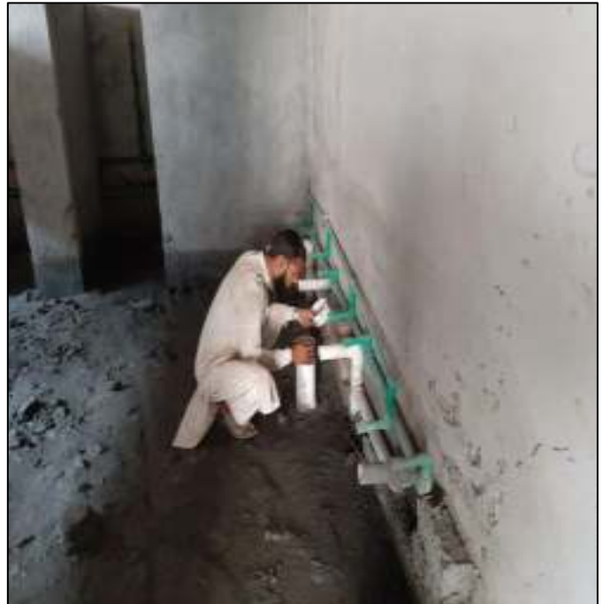
Picture 59: Plumbing work in washrooms at 5 th floor
